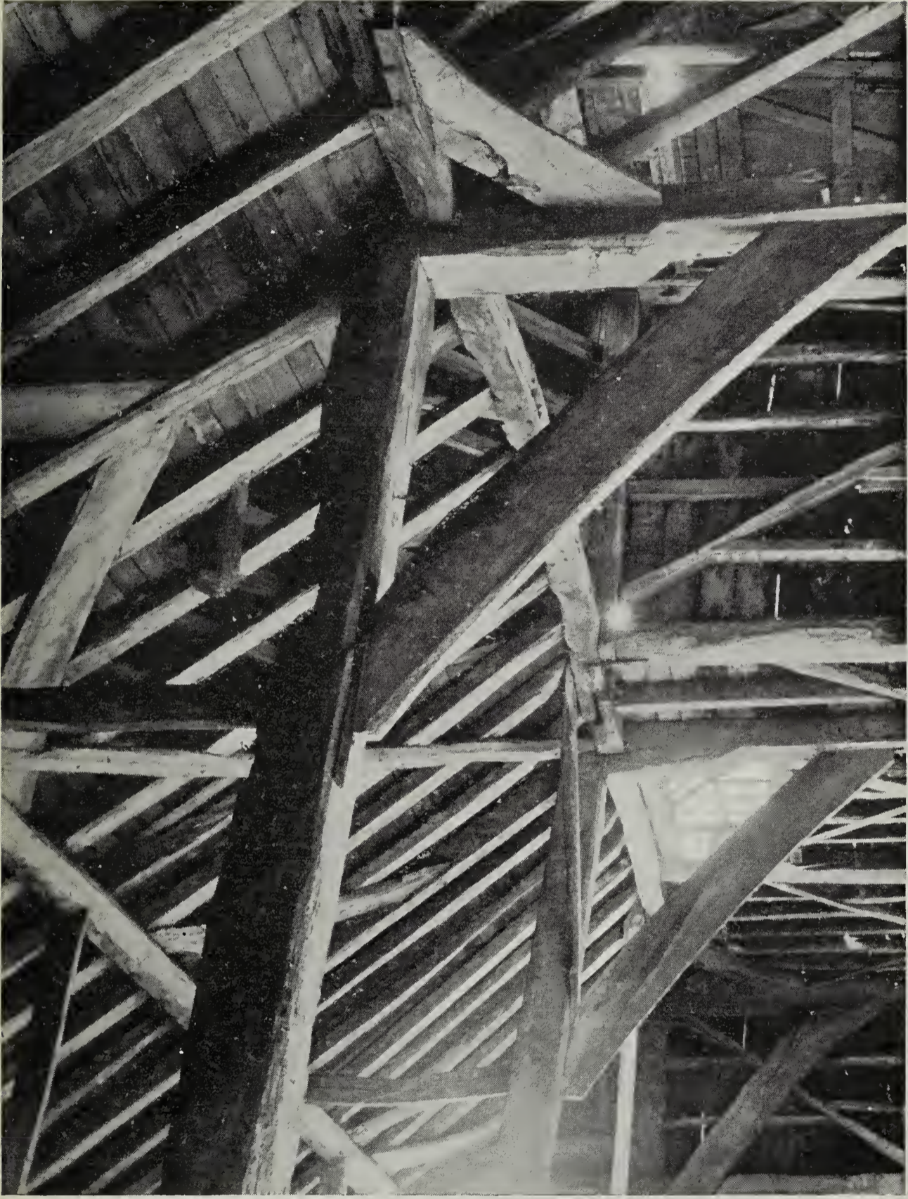
THE CRACKED BEAM OF THE SHIP
